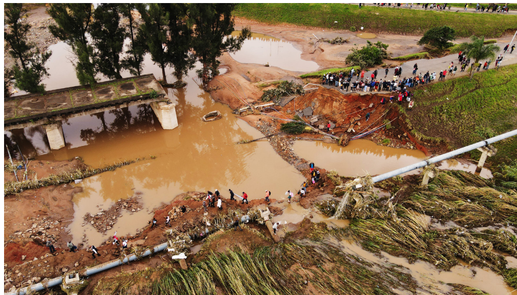
Flood damage in the province of KwaZulu-Natal, following the floods of April 2022, the most catastrophic recorded natural disaster in South Africa's history. Credit: Shutterstock
