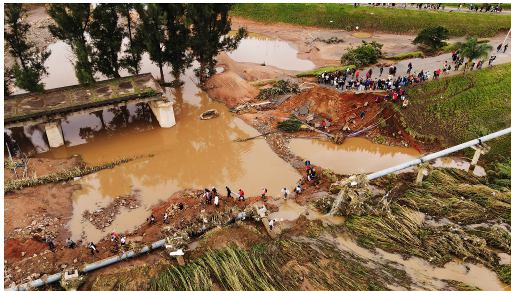
Flood damage in the province of KwaZulu-Natal, following the floods of April 2022, the most catastrophic recorded natural disaster in South Africa's history. Credit: Shutterstock
