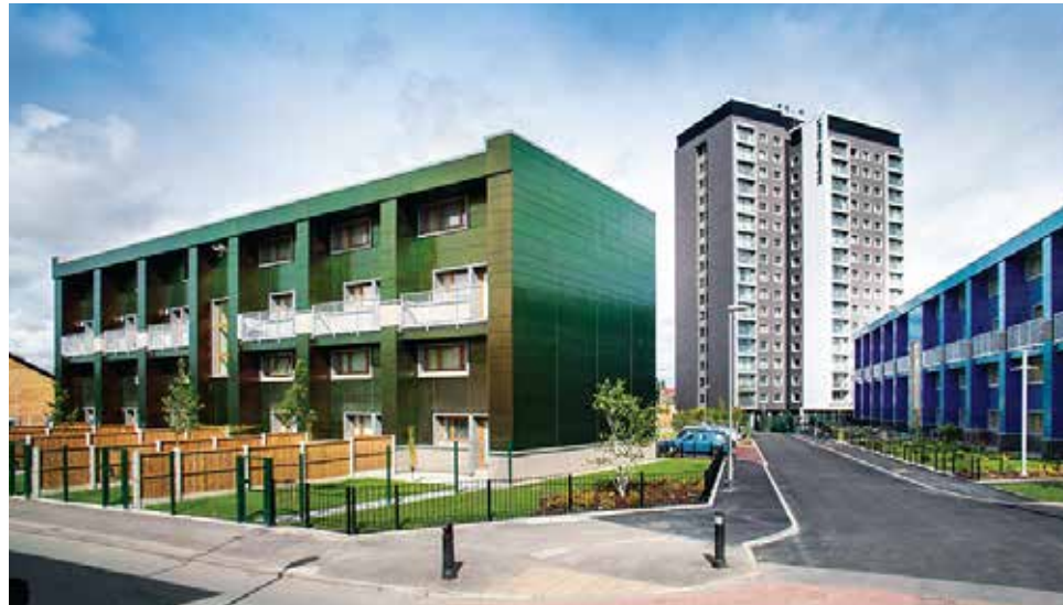
Deep energy retrofit of Erneley Close, by Manchester City Council, an exciting example of a regeneration project in the UK. Nominated for a Passivhaus Award. Photo: Tim Bradley Photography
