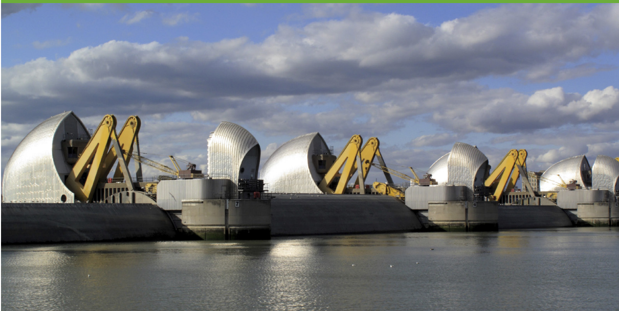
Figure 7. The Thames Flood Barrier with its gates closed to protect against a storm surge
