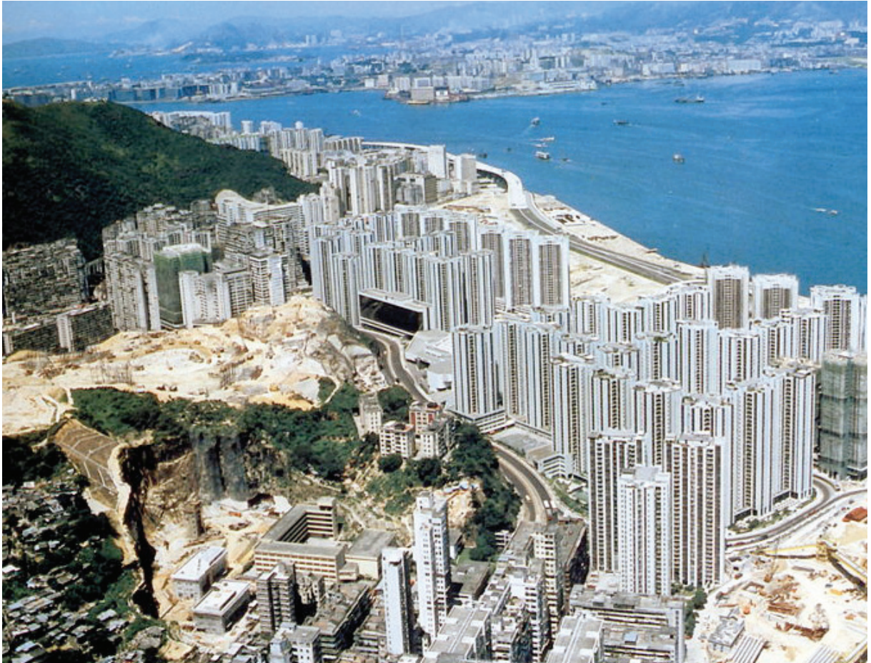
Figure 65: Taikoo Shing under construction, 1980s (Source: WiNG, published under Creative Commons)
