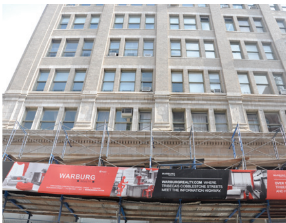
Figure 34: Former industrial buildings awaiting conversion, adaptation and/or redevelopment, 2011 (Source: Juliet Davis)
