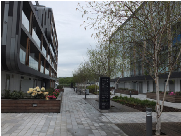
Woolwich Central, Woolwich
