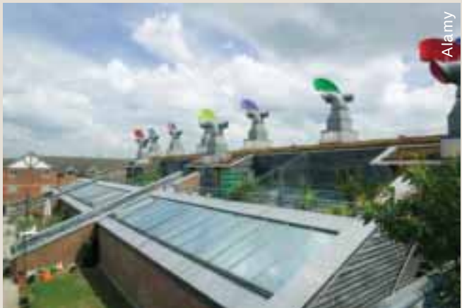
BedZED (Beddington Zero Energy Development), London
