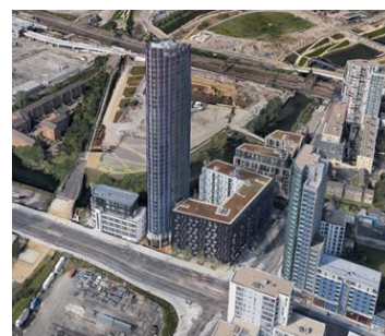
Stratford Halo 43-storey blue-and-purple clad tower on Stratford High Street, surrounded by lower blocks.
