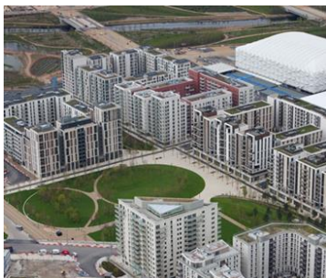
East Village Mid-rise courtyard blocks, built as Athletes' Village for 2012 Olympics.
