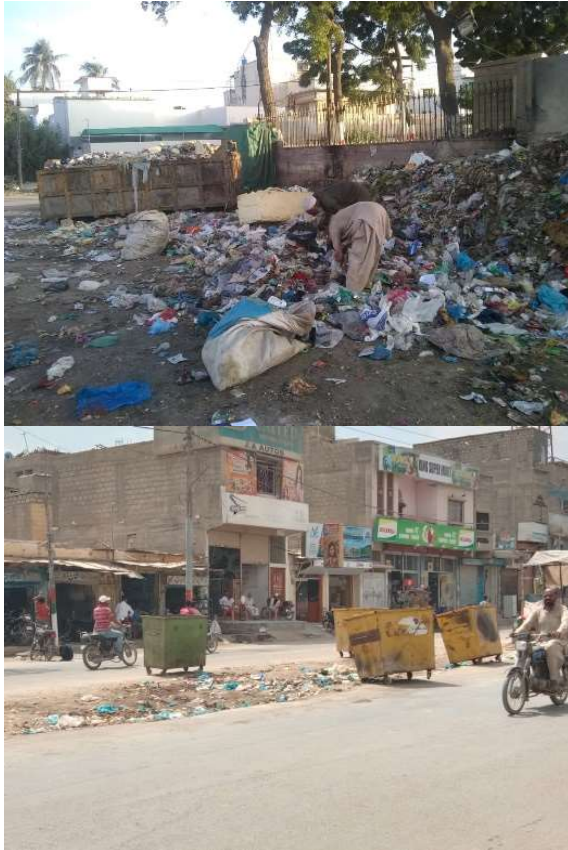
Figure 9. Waste bins and Containers installed by SSWMB functioning as Katchra Kundis.
