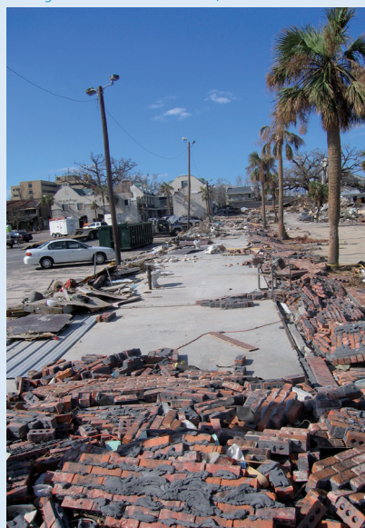
Damages from Hurricane Katrina, © Munich Re
