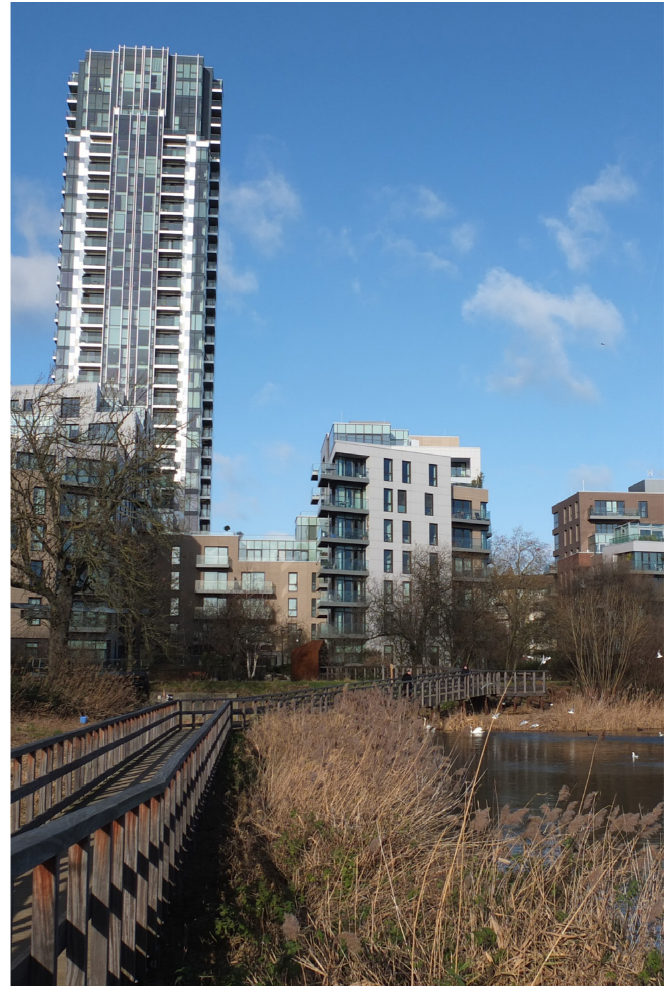
Looking across the reservoir and wetlands at some of the buildings of Woodberry Down, whose master plan weaves in green space.
