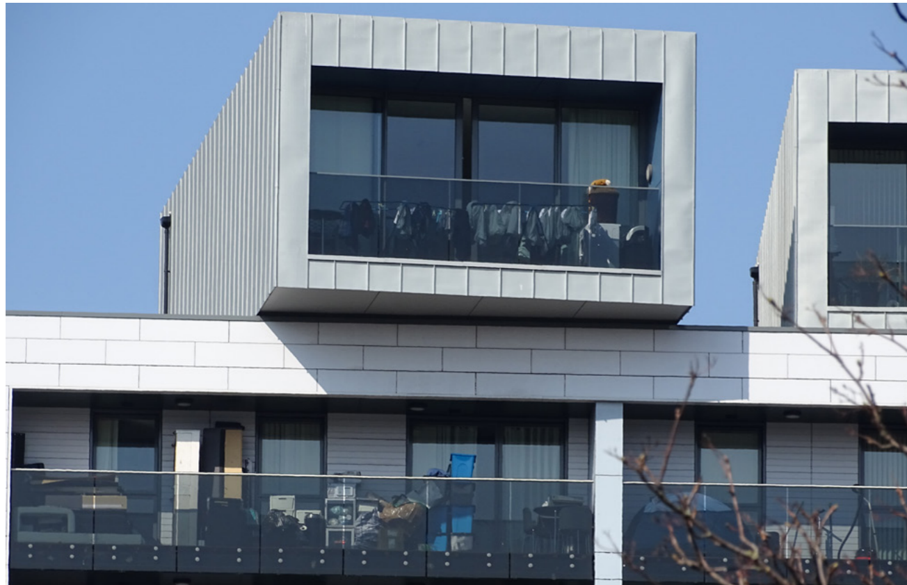
Upper floors of Thurston Point. Note the belongings stored on the balconies.
