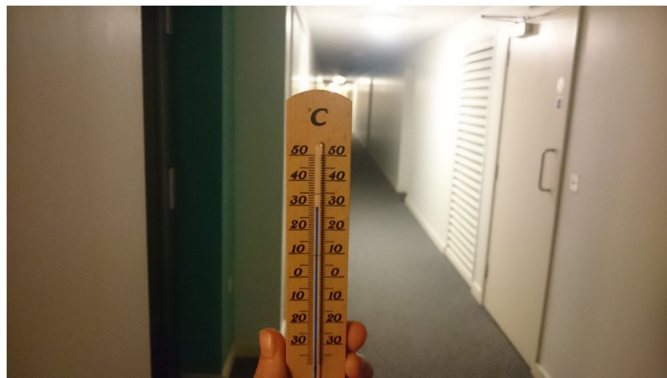
Resident's photo showing internal temperature of corridor at Greenwich Creekside (Autumn 2017)
