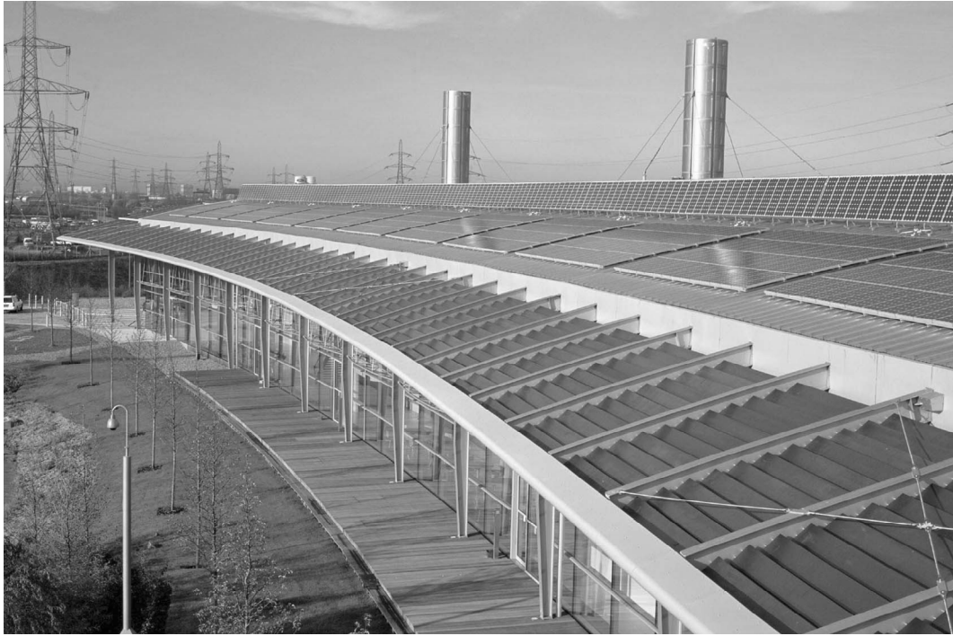
Figure 6. An example of the modern building design to help to reverse the trend towards sustainable development
